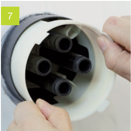
Remove assembly pipe
