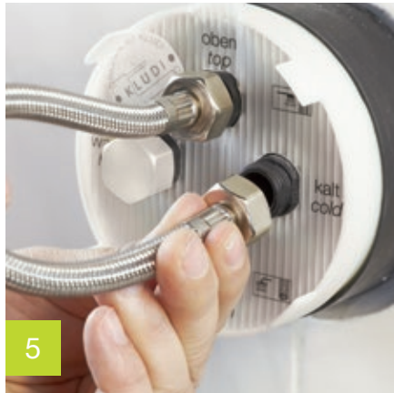
Flush in accordance with DIN 1988 using integrated flushing set – without opening the box
