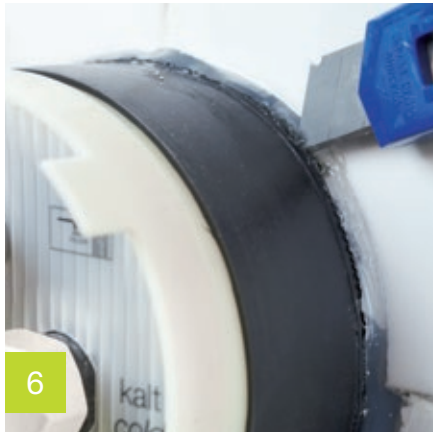
Trim to size – the inside of the box remains protected from dirt during the entire construction phase
